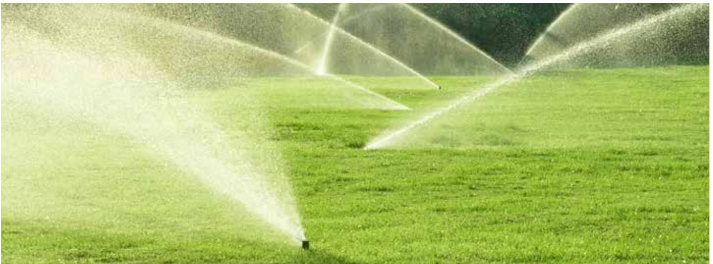
Automatic garden sprinkling system
